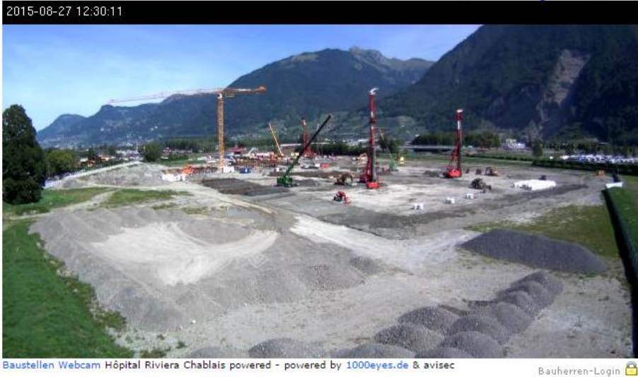
Figure 17: Final decision to use vibratory compaction to reduce the liquefaction risk
