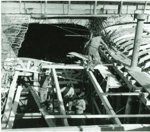
Figure 6. Left: Construction of the main beams and arched slab at once. Right: Cross-section of the main beam over a pillar.
